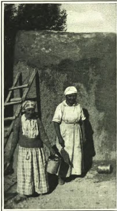
ALVINA AND LUCIANA READY TO PLASTER
