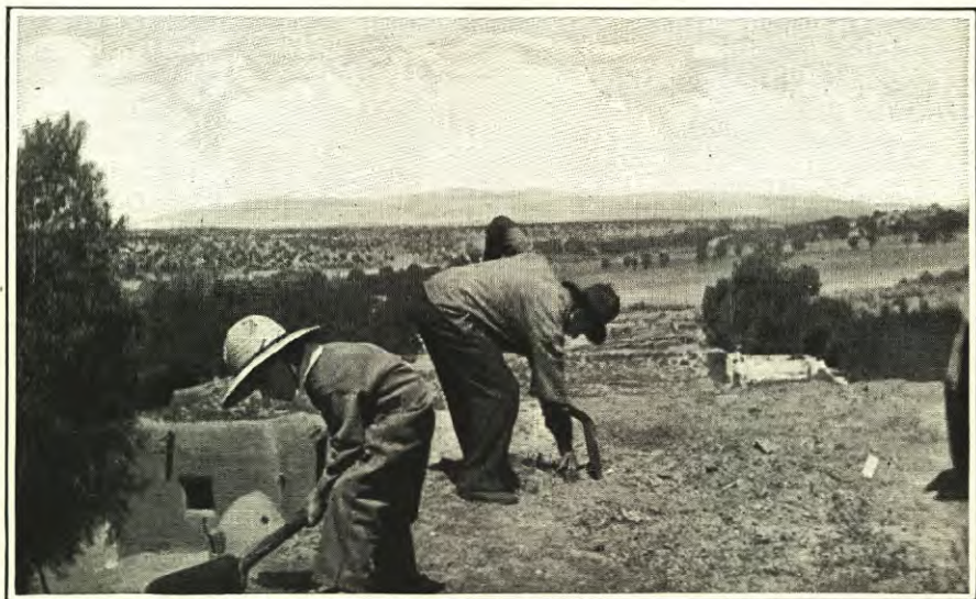
SHOVELING DIRT OFF THE ROOF
