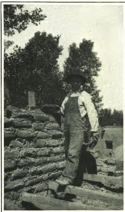
DEMOLISHING THE KITCHEN WALL
